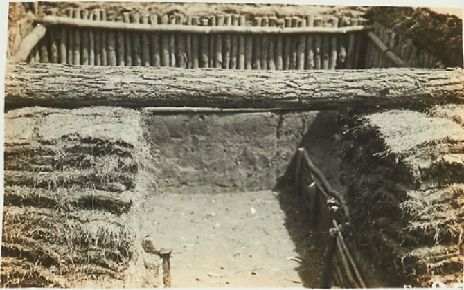
HOSPITAL IN TRENCH
